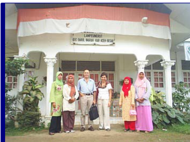
One of the health centres rebuilt as part of emergency project in Aceh-Indonesia.
